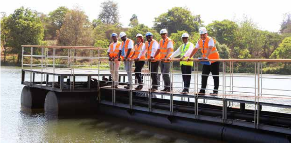
The Pontoon as installed on site
