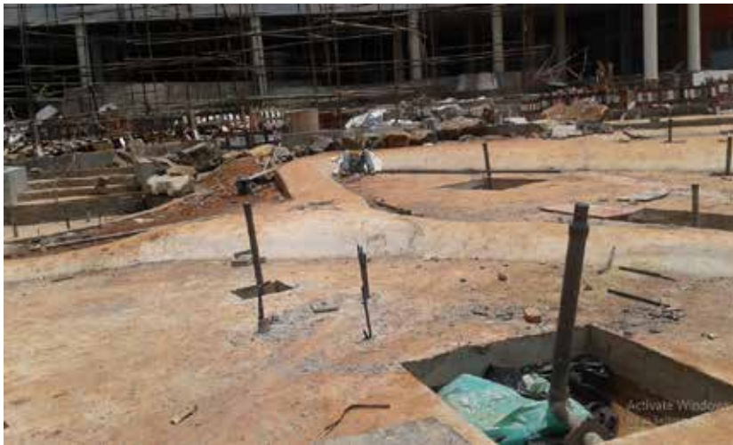
Water play area under construction
