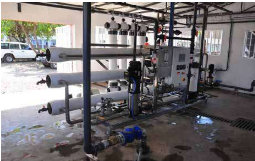
Completed Installation on site
