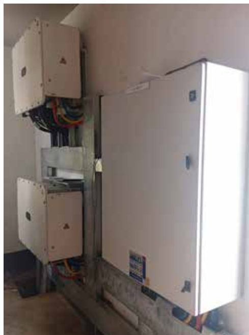
Installed Site Pictures
